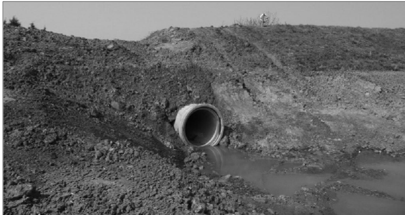
Figure 4. Pipe at reservoir number 8
