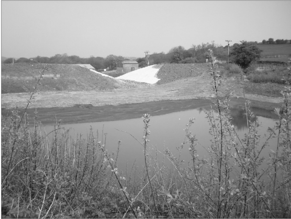
Figure 1. Concrete weir in centre of embankment of reservoir number 3.
