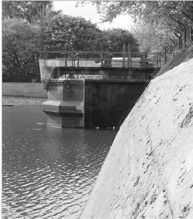
Figure 2. Overflow shaft of reservoir number 2.
